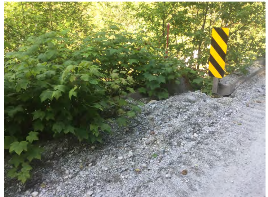
Left Approach Upstream Fender
