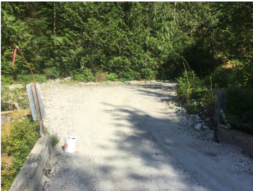
Left Approach Facing Away From Bridge
