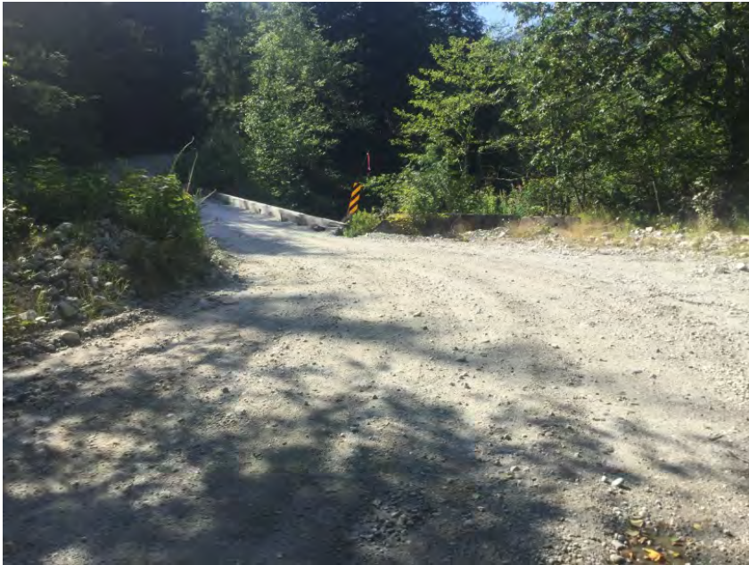
Left Approach Facing Bridge
