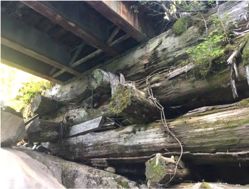
Left Bank Abutment
