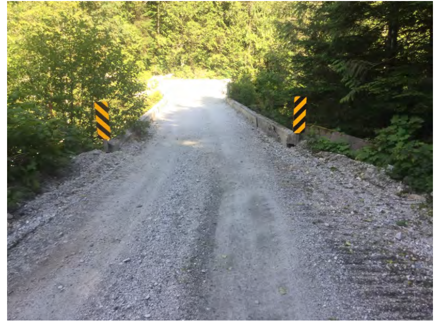
Right Approach Facing Bridge
