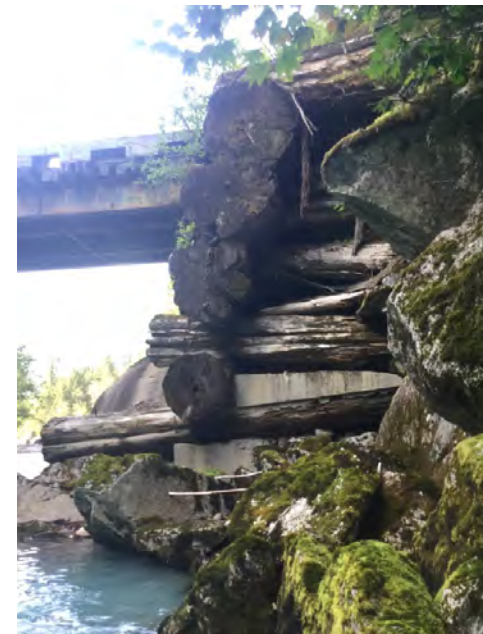
Left Abutment Downstream Corner
