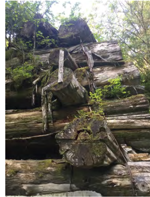
Left Abutment Downstream Corner
