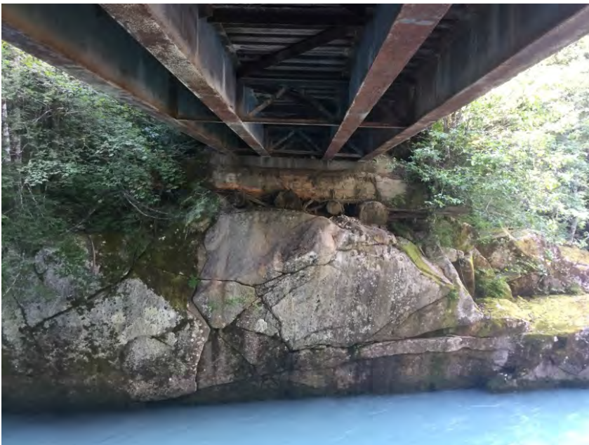
Right Bank Abutment
