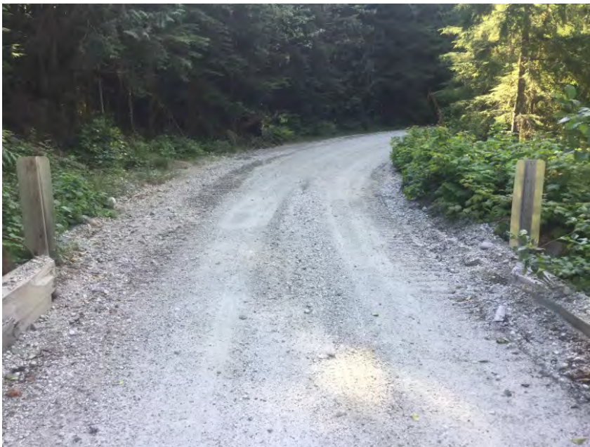
Right Approach Facing Away From Bridge
